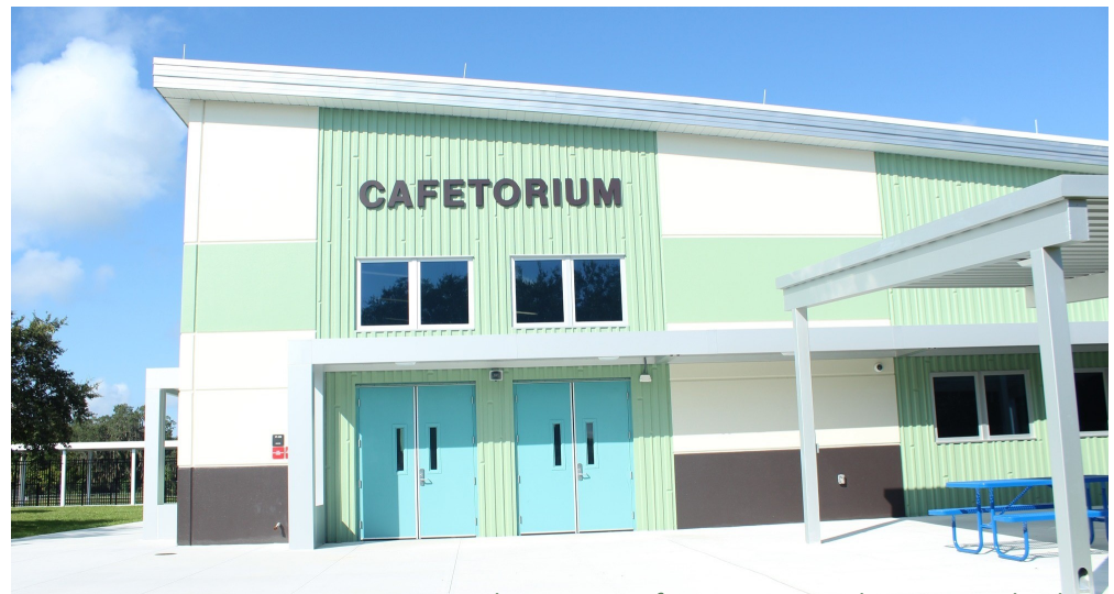
Photo: New Cafetorium, Mims Elementary School
